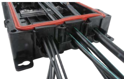
Various cable installation
